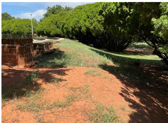
Figure 2: Amphitheater access without sidewalk.
