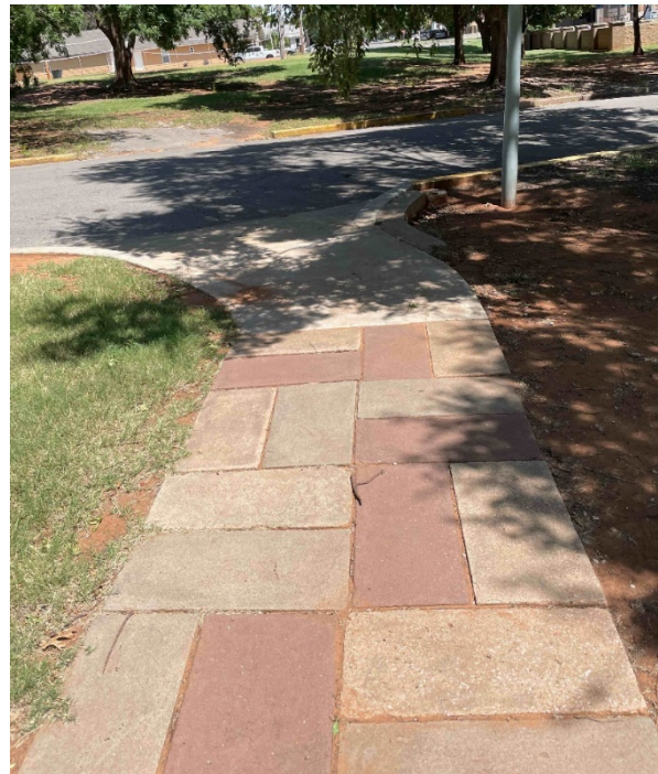
Figure 3: Existing Paver Sidewalk from Amphitheater
